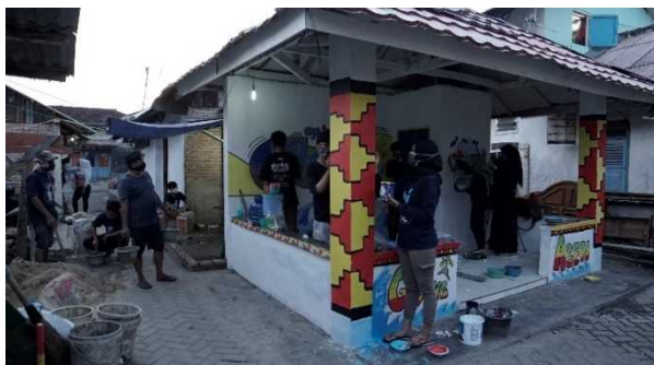
Repairs and painting of the facility
