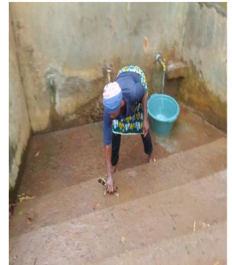
A beneficiary cleaning the water supply facilities
