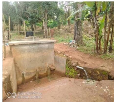
Water supply facilities completed under this project
