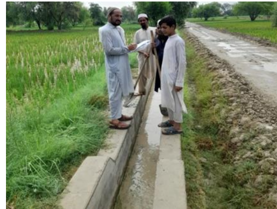
Irrigation canal after implementation
