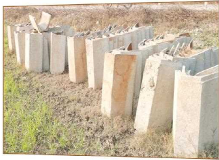
Storage of concrete irrigation channels
