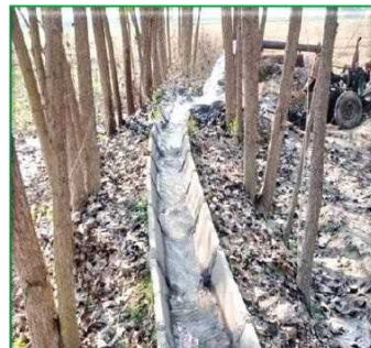
Preventing wastage with water flowing in a concrete channel
