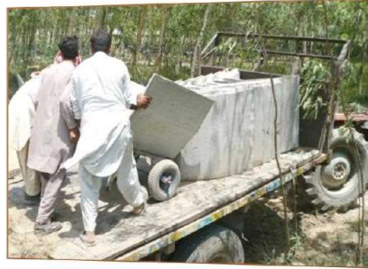
Transporting concrete irrigation channels
