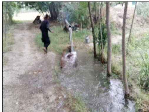
Water wastage on both sides of a muddy, unlined channel.
