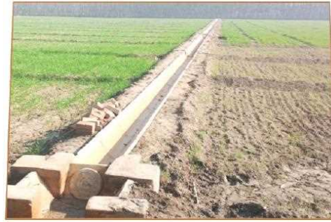
Constructing concrete irrigation channels
