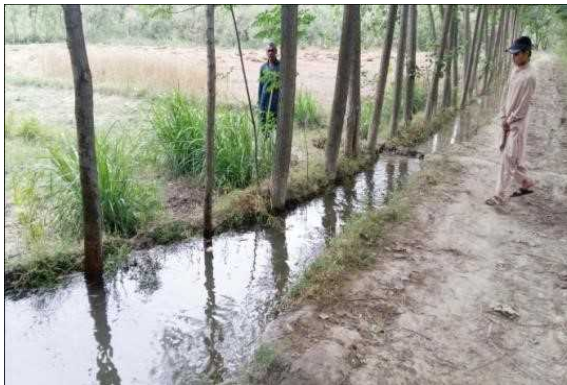
Current view of unlined water course
