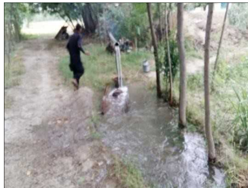
Current situation of water wastage on both sides of muddy, unlined channel.
