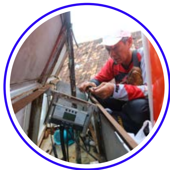
Monitoring & Evaluation public toilet and effectiveness the infrastructure after 5 years
