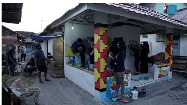
Repairs and painting of the facility
